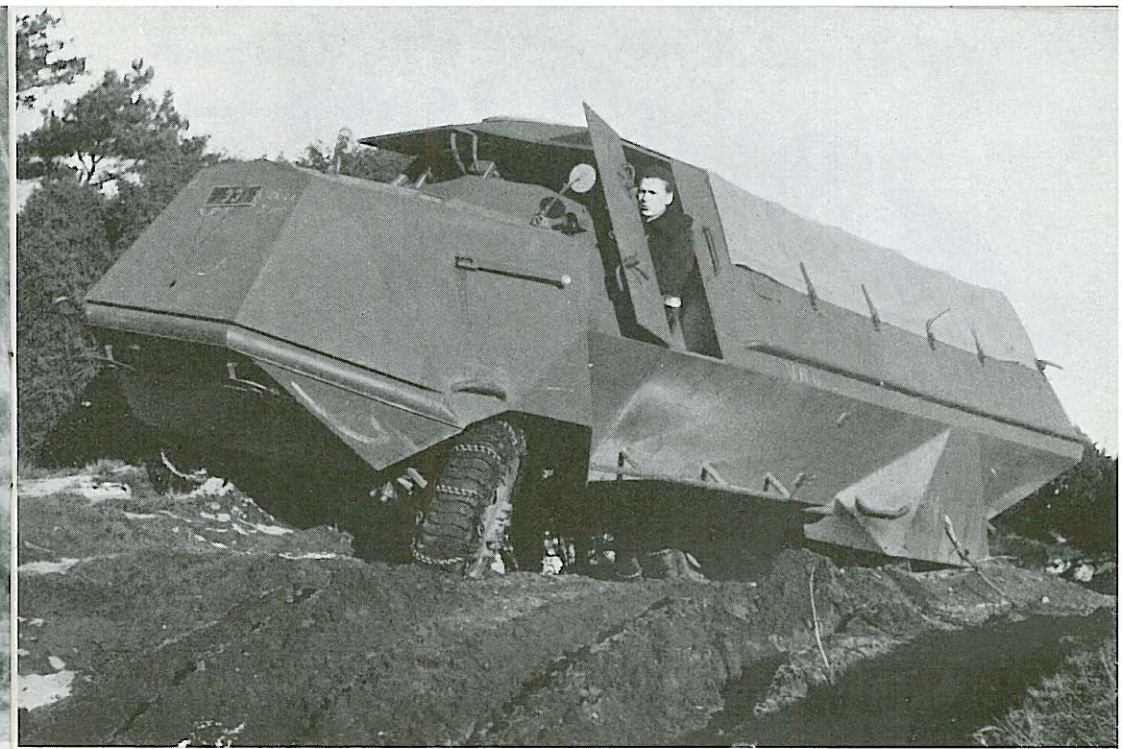
The TLV 4-wheel-driven, cross-country truck with armoured body was another.
